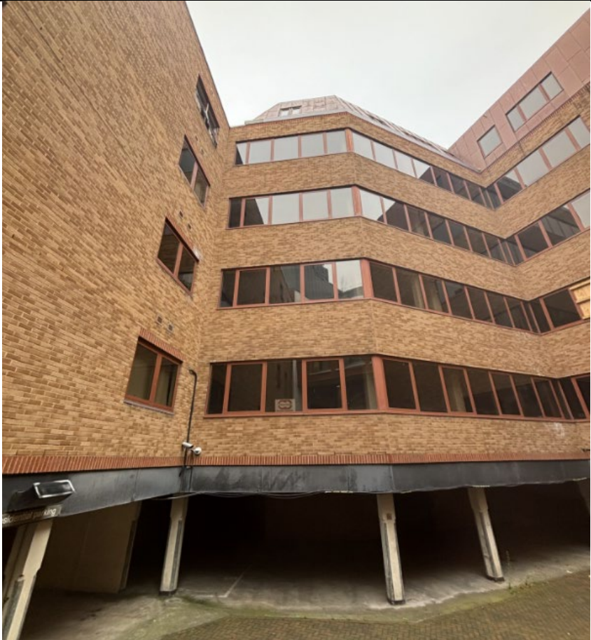
View of building from rear courtyard
