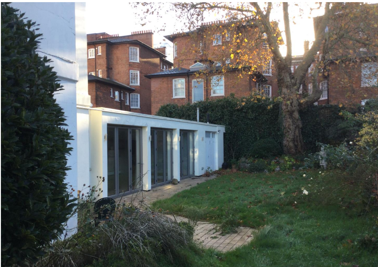
View from garden of property showing existing rear extension
